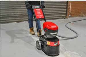
Grinding Concrete
